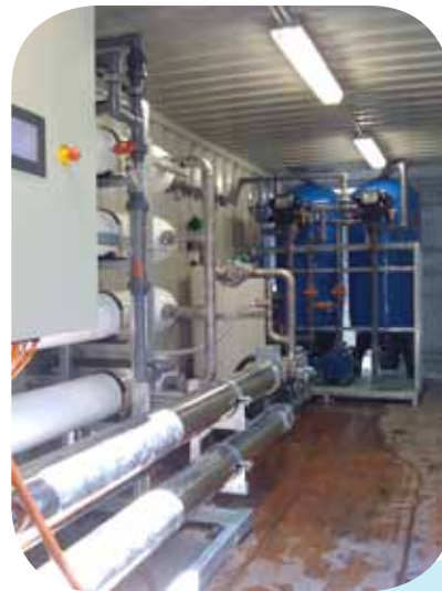
Fully automated Sea Water Reverse Osmosis Plant
