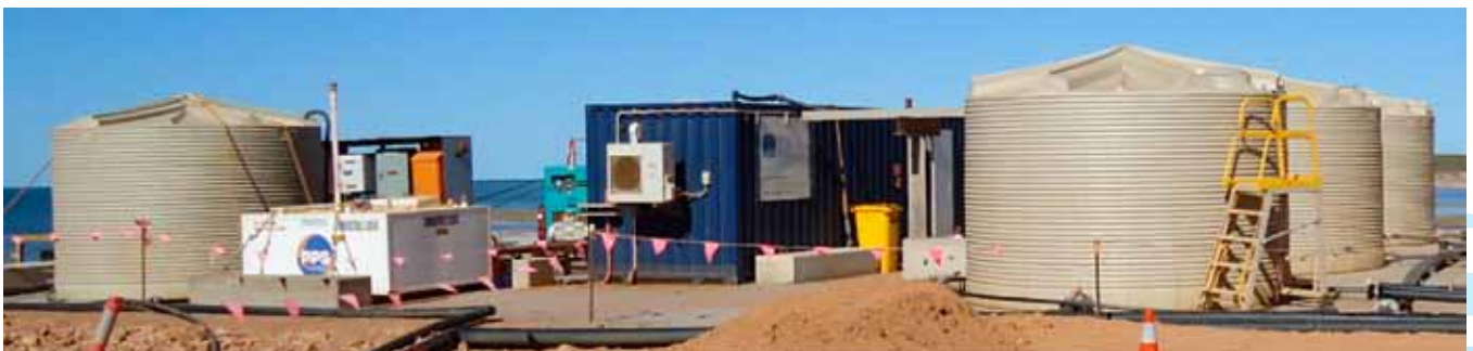
MAK Sea Water RO Unit – Part of Chevron's Gorgon project. Water Systems and operation management by MAK
