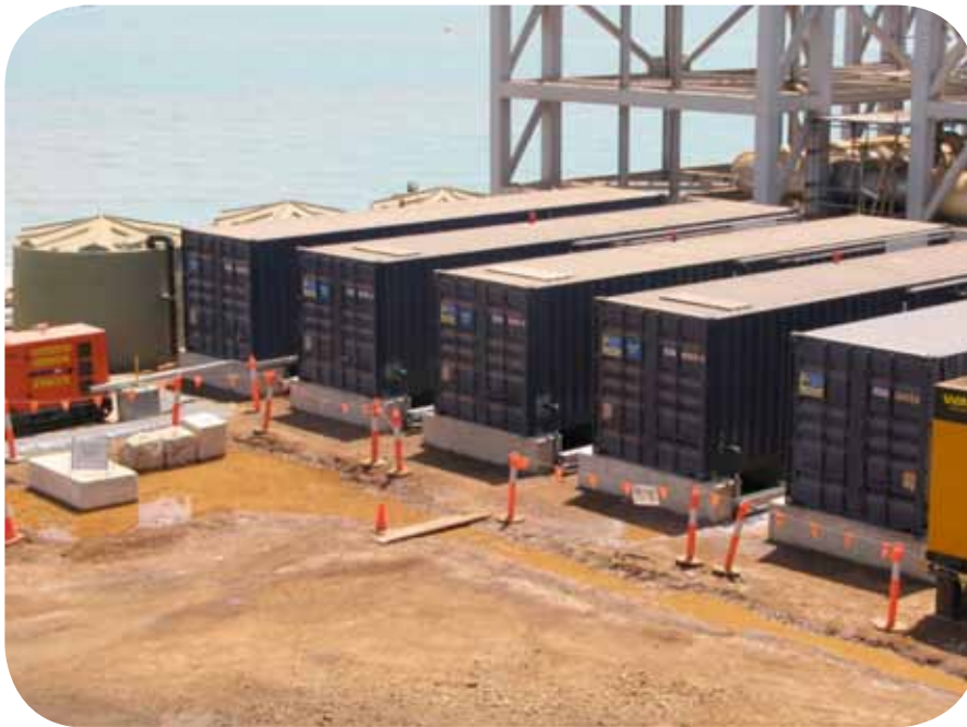
Five MAK 200m 3 /day Sea Water Reverse Osmosis on hire in Karratha WA
