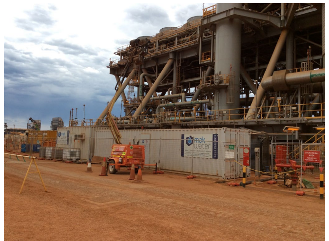
The Brackish Water Reverse Osmosis hire plants on site on Barrow Island
