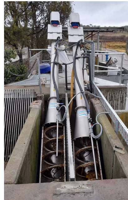
Installed new screw screens
