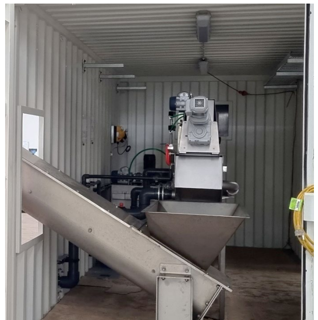
Internal view of the plant under construction in MAK Water factory
