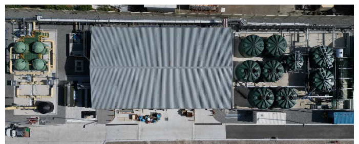
Overhead view of treatment plant
