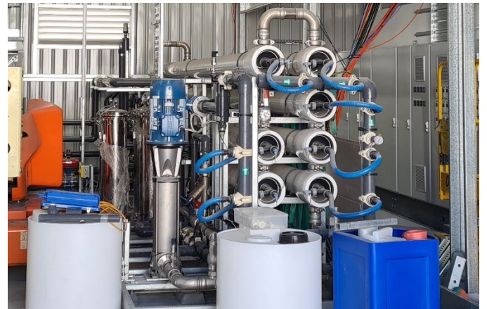
Reverse Osmosis (RO) skid & small chemical containers during construction
