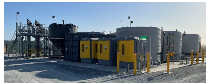
External view of plant
