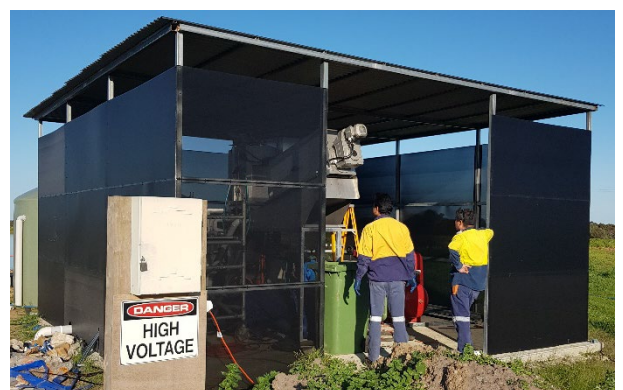
Installing the protective enclosure
