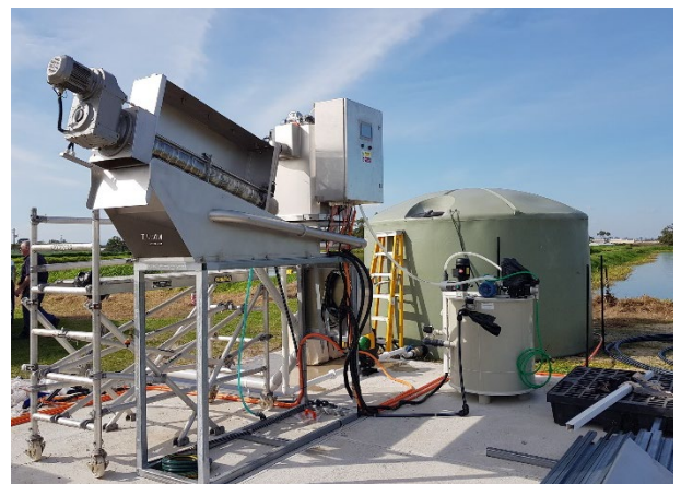
DSP and ASP during installation, prior to erection of protective enclosure
