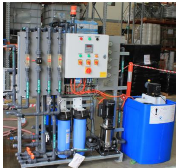
BWROB Water Treatment Plant
