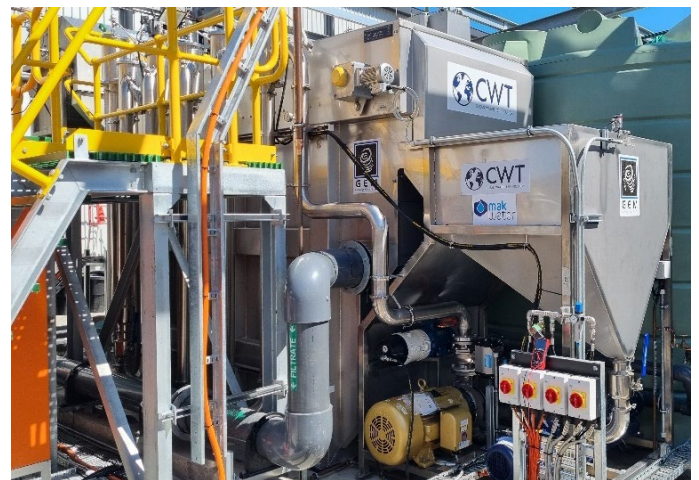
GEM-DAF and access platform during installation on site.
