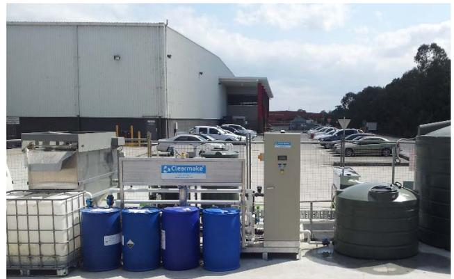
*The dissolved air flotation system and oil water separator on site*
