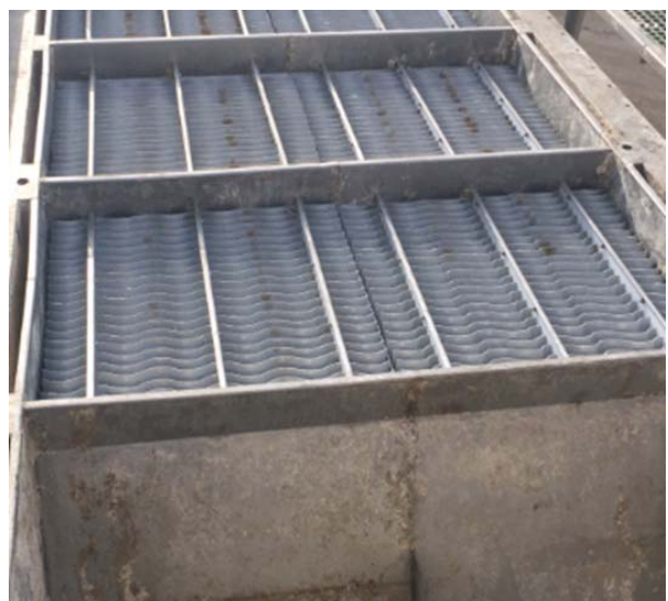
New installed plate packs in DAF
