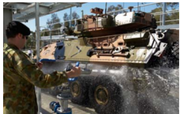
The dissolved air flotation wash bay water recycling system in use at the Enoggera Barracks
