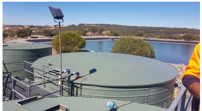
New upgraded colour matched Roofs
