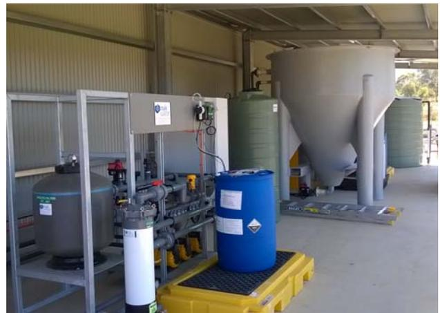
*Water recycling system capable of treating 5,000 litres per hour of wash water*
