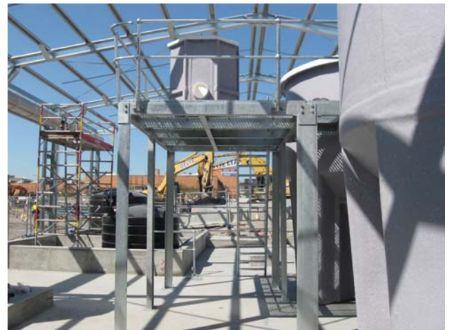
Installation of the Gravity Clarifier on site for the Clem7 Tunnel
