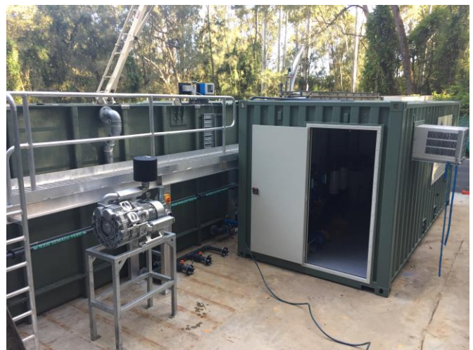
MAK Water MBBR plant on-site installation
