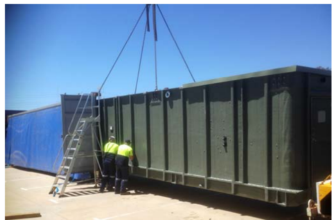
MAK Water's ASBR plants fit into standard shipping containers for mechanically protected, low cost sea freight
