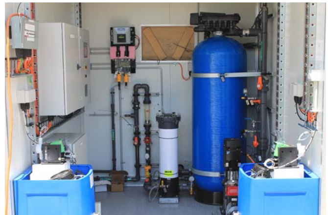
Containerised MMF plant for plug-and-play installation
