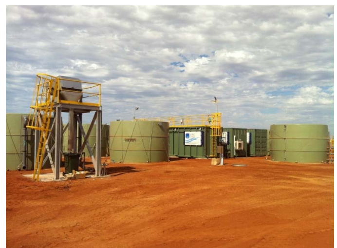
Waste Water Treatment Plants on site in Onslow
