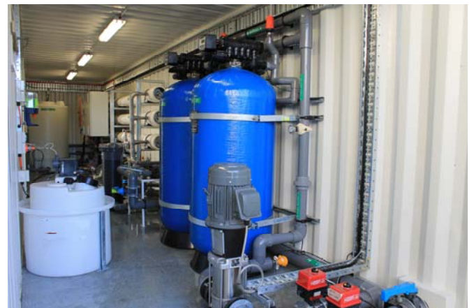
Sea Water Reverse Osmosis Plant undergoes factory acceptance testing
