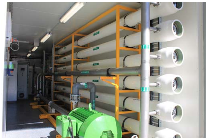
The Sea Water Reverse Osmosis Plant undergoes Factory Acceptance Testing
