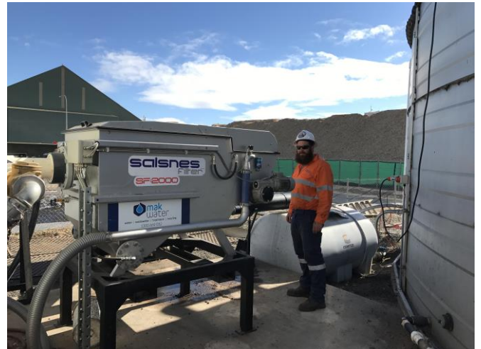
MAK Water provided all site installation works
