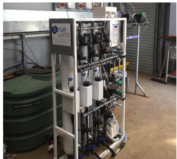
MAK Water UF-B's are able to treat a wide range of highly variable waters with <50 NTU of turbidity and <100 mg/L of suspended solids
