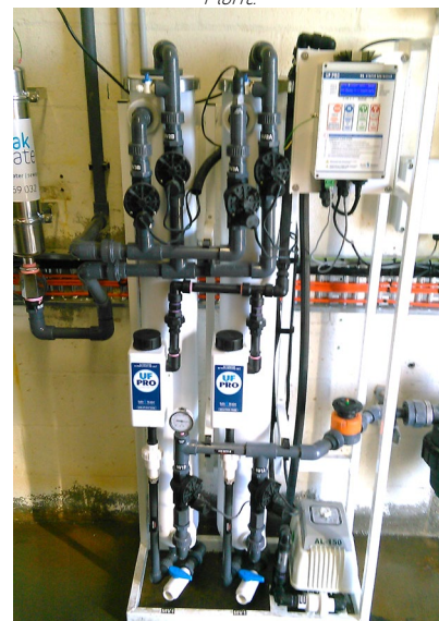
40 m 3 /Day UF/UV Potable Water Solution
