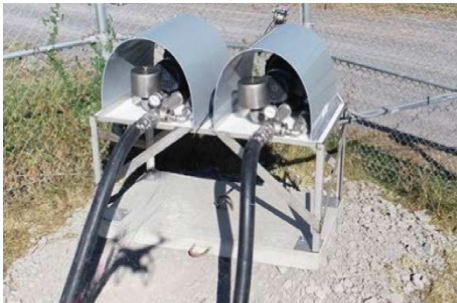
Lagoon Master Aerator V2 with shore mounted blowers
