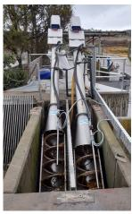
Machine carpentry, drive guard and anti-wear material on screw in 304L SS, bolts A2 (304 SS) (standard)
