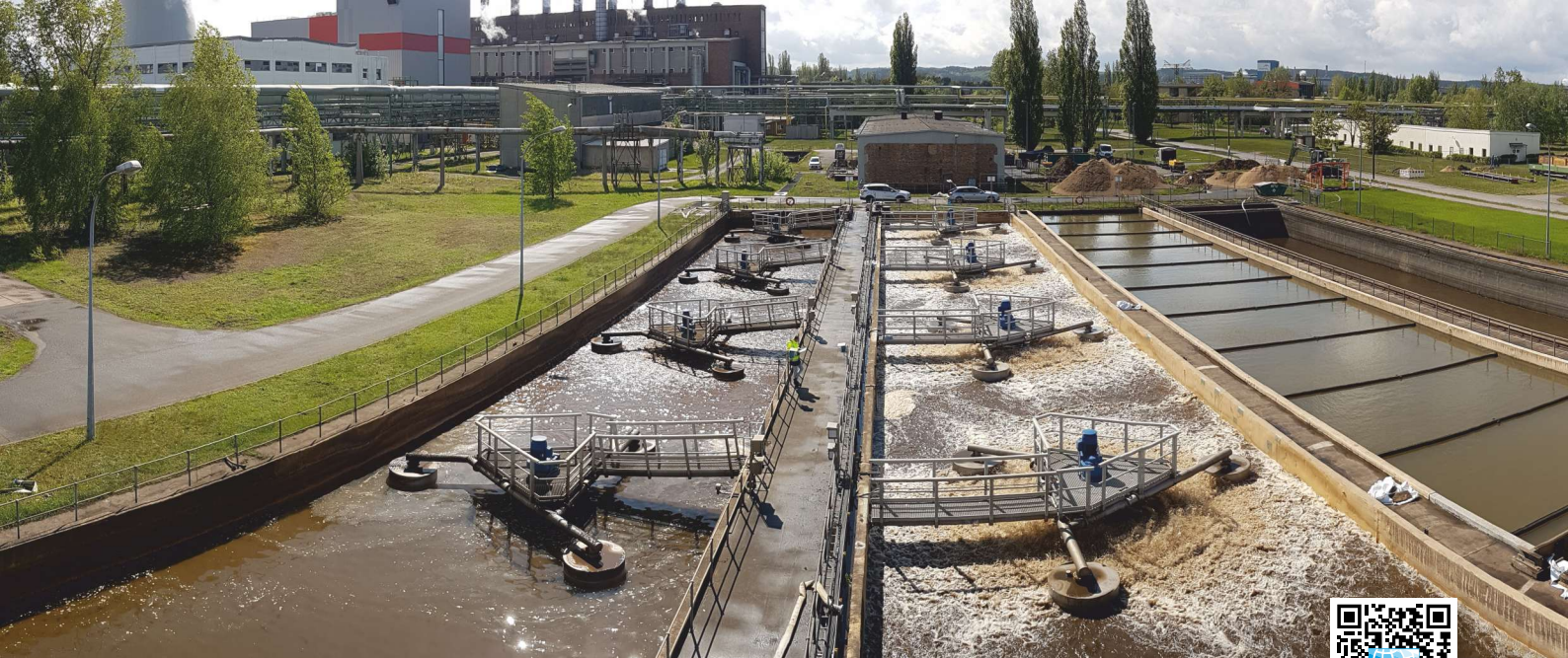
Floating BSK®-Turbines Ø 1,600 mm installed in a German wastewater treatment plant
