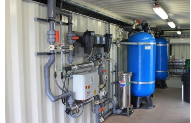
MAK Containerised 300 m 3 /day MMF Plant
