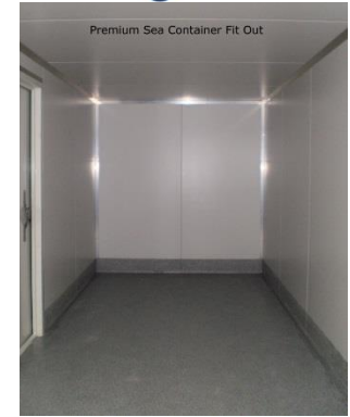
Premium Fit Out (insulation, floor coating and access door)
