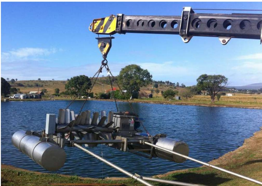
Figure 9. A fully assembled Floating Brush Aerator (without Splash Shields) being lifted/installed into a lagoon
