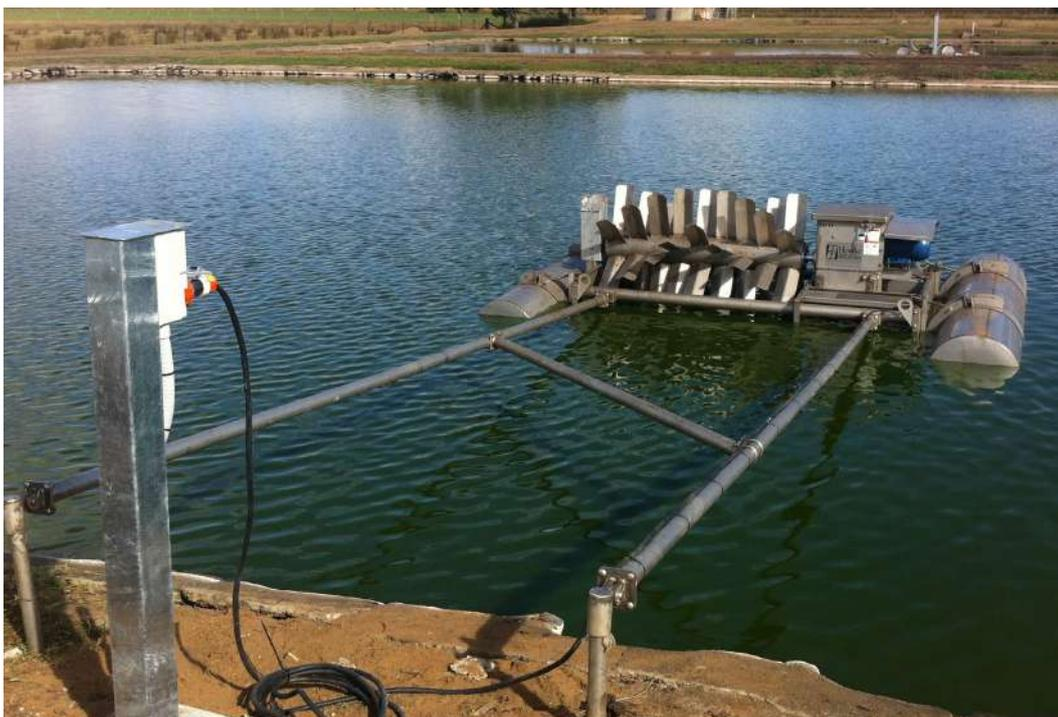
Figure 11. Completed installation of a Floating Brush Aerator (without Splash Shields) at a municipal lagoon plant in QLD
