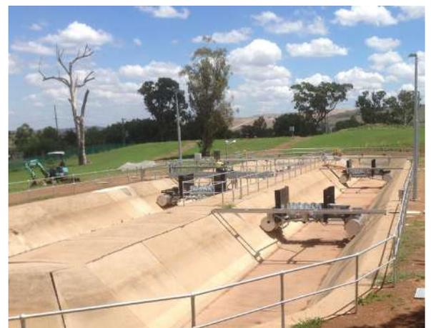
Figure 3 & 4. Floating Brush Aerators with Splash Shields in a Pasveer ditch
