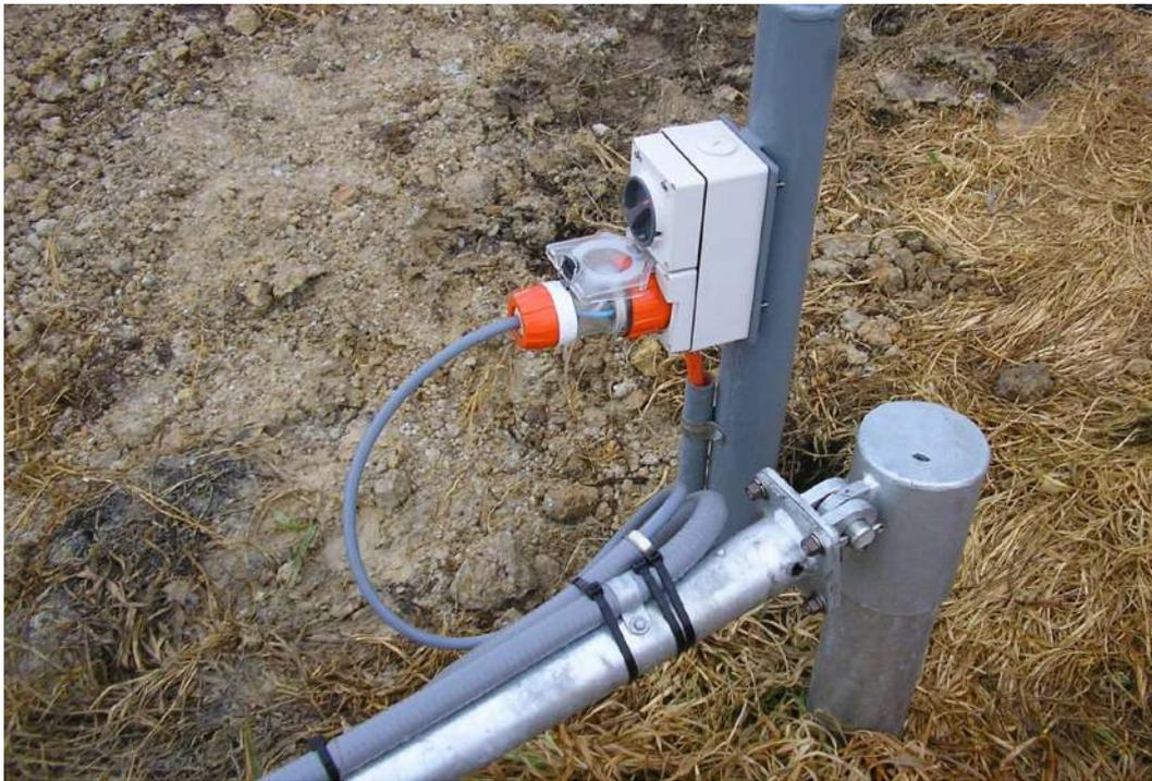
Figure 10. 3-phase electrical socket with local isolator mounted on post.
