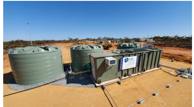
MAK Water modular ASBR plant installed onsite
