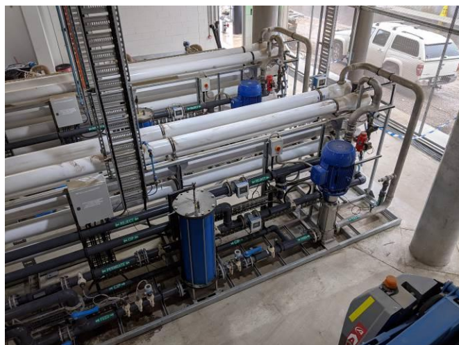
Two stage Reverse Osmosis (RO) configuration with 75% recovery rate
