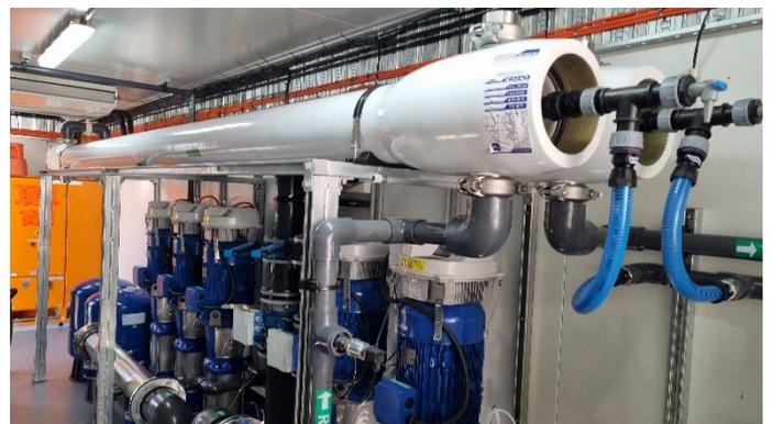
*Internal view of the containerised BWRO plant*
