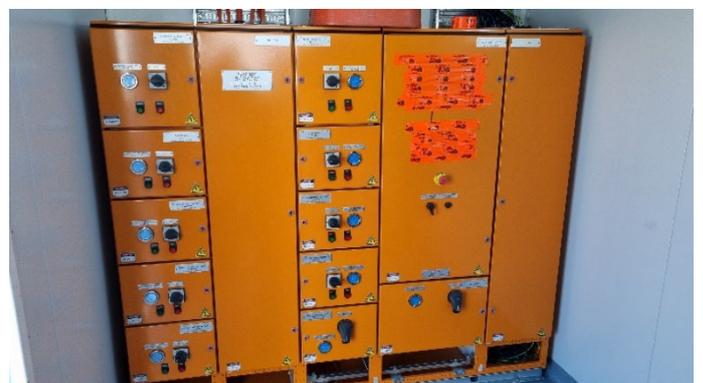
*Form-4 mine-spec control panel to client specifications*
