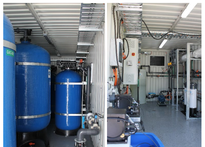
Internal views of the containerised MMF and BWRO plants
