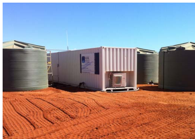
Brackish Water Reverse Osmosis plant on site
