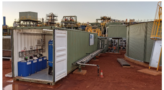
MAK Water containerised BWRO plant installed onsite
