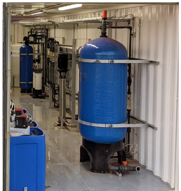
Internal view of the containerised BWRO plant
