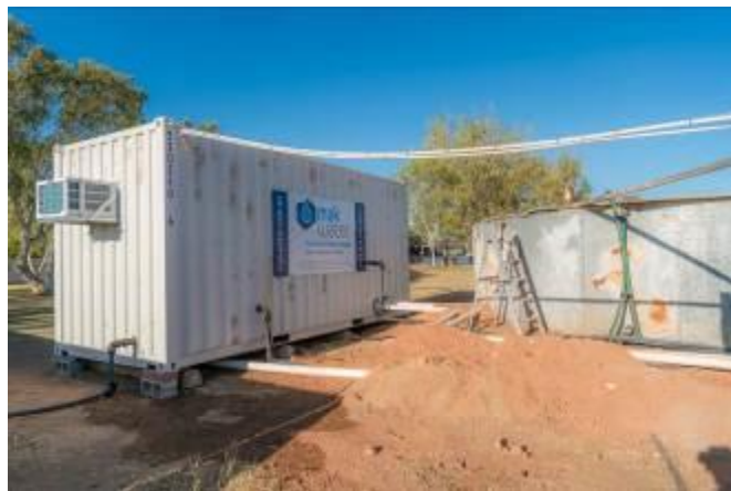
Containerised Brackish Water Reverse Osmosis plant installed onsite
