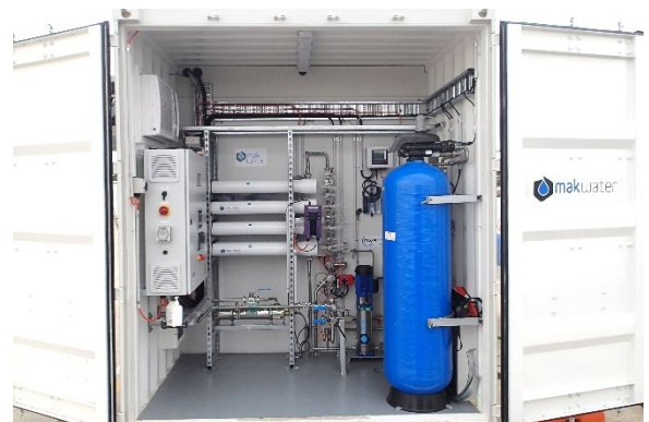
BWRO 030 system integrated with MAKPAK deionisation
