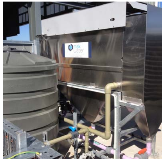
The dissolved air flotation plant on site
