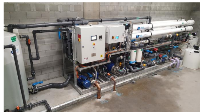
Fully commissioned BWRO Plant on-site in the Gold Coast, QLD
