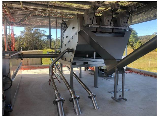
*Dewatering Screw Press DSP-403 installed.*
