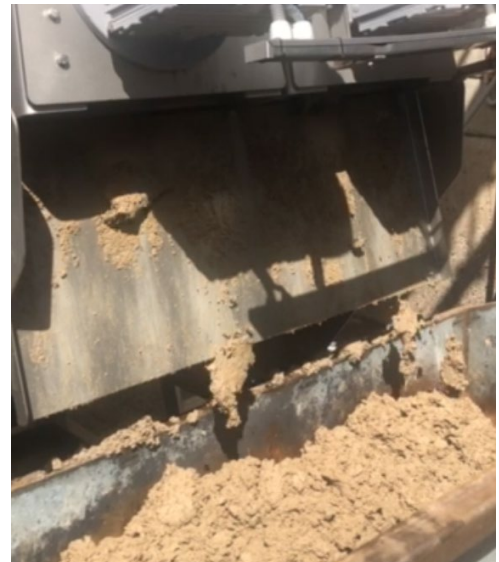
Dewatered sludge exiting DSP via chute
