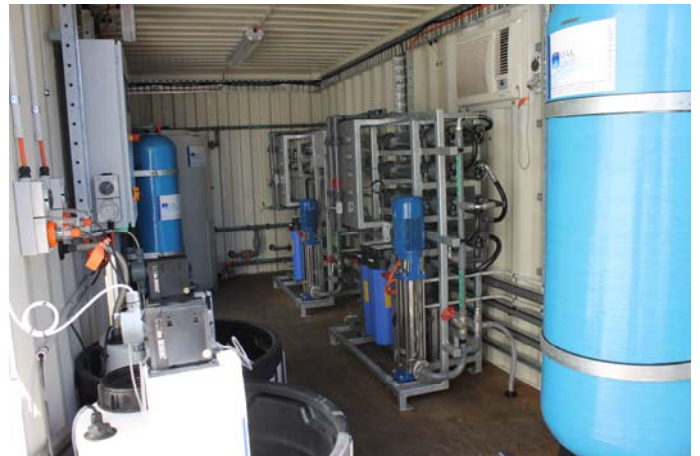
Containerised two pass reverse osmosis plant
