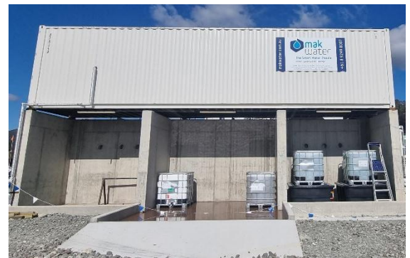
Containerised Filter Press mounted on top of concrete bunker for dewatered cake storage & collection
