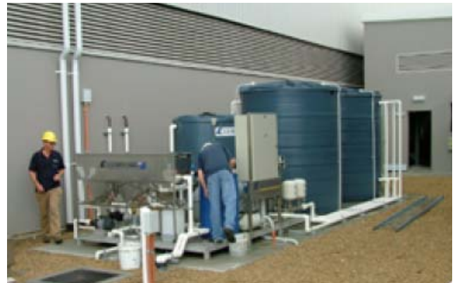
The gravity clarification system and oil water separator
