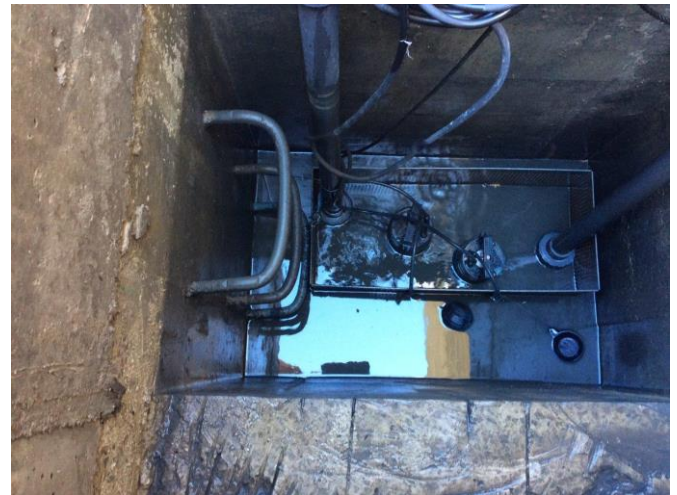
Perforated Mesh Screen in Pump Pit
