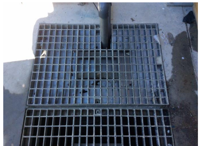
Perforated Mesh Screen at Pit Covers
