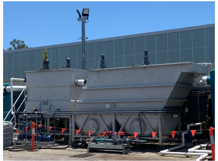
MAK Water Lamella Clarifier installed onsite
