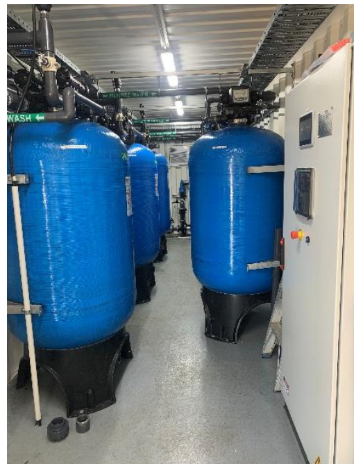
Internal view of the containerised MMF plant
