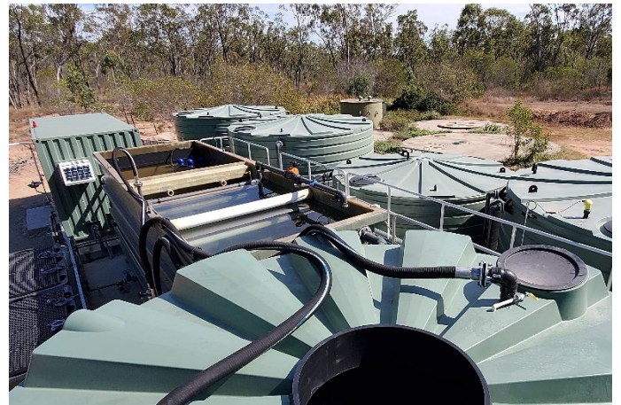
FRP Tanks, MBBR+ and MMF containerised plant
