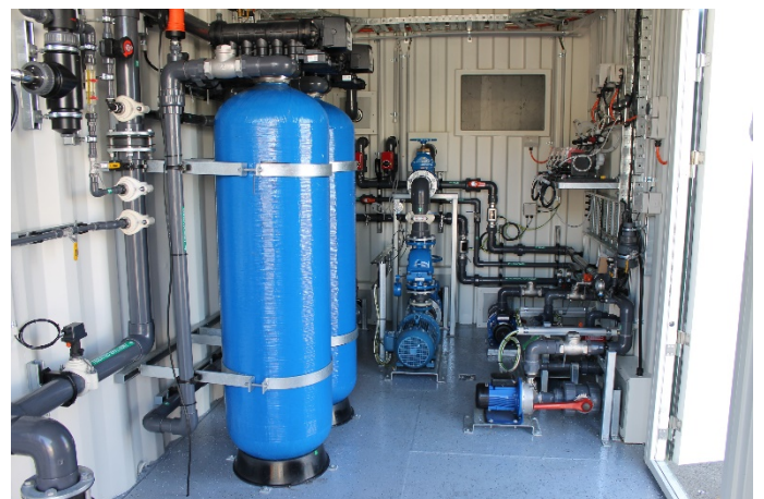
Inside containerised MMF plant
