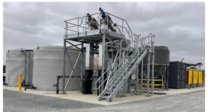
Left to right, Balance tanks, Influent Screens on custom elevated platform, Sludge Tank, 40' containerised plant room, self-bunded chemical storage & dosing cabinets.
