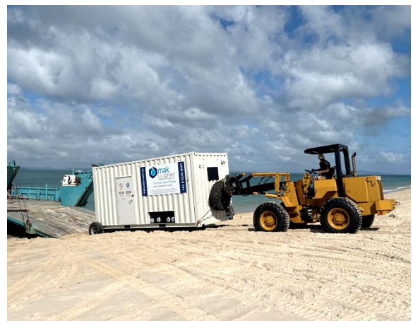
STP being unloaded
