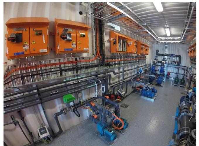
Inside MAK Water containerised MBR+ pump & control station
