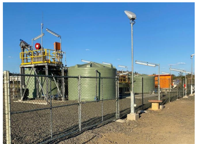
Site photo showing scale of installation with storage tanks, MBR+ reactor, pump & control container and elevated work platform
