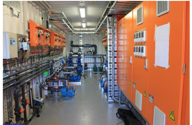
Modular designed plant fully assembled, and factory tested
